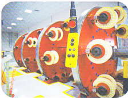
ISO 8 CTC Insulation Department
